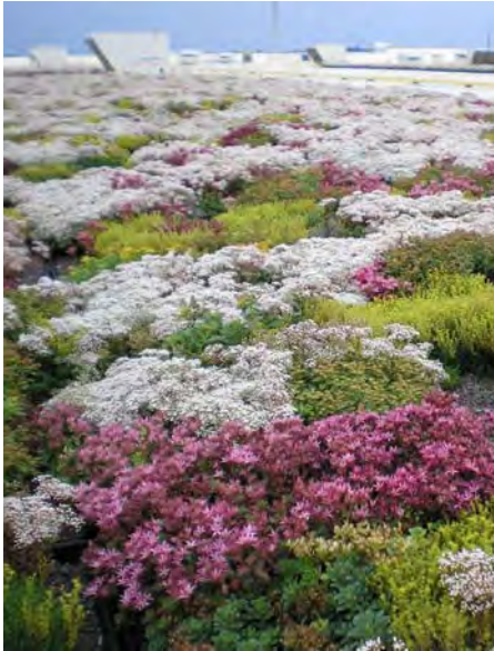
Figure 9. Vegetative Roof after 1 year of growth
