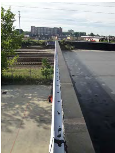
Figure 8. View from the maintenance roof looking at the commuter/freight/passenger rail
